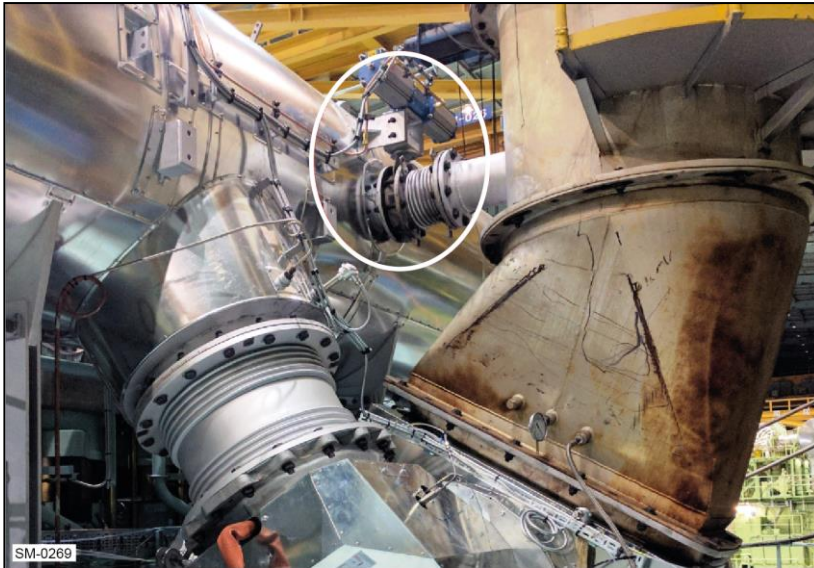
Figure 2-23: Exhaust gas waste gate installation
