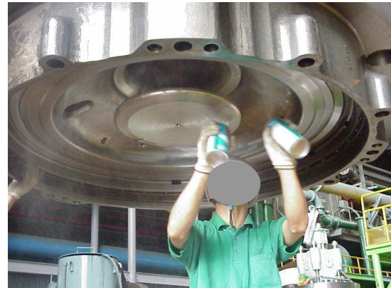
Combustion chamber after cleaning.
